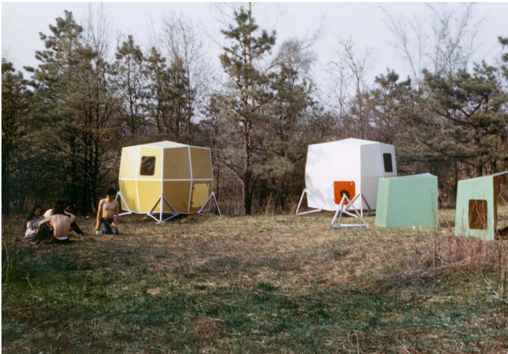
Ken Isaacs, 8' Microhouse installed on-site with assembled tetrahedron legs, c. 1972. Photo courtesy the artist
